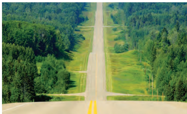
Figure 3.23 Road construction often causes habitat fragmentation.
